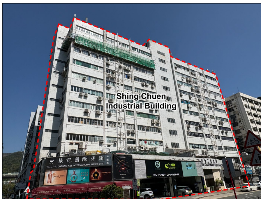
Photo 1.1 Existing Photo of Shing Chuen Industrial Building
